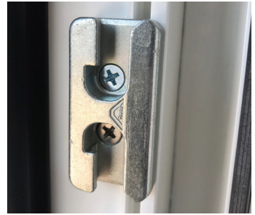
Figure 5: Mushroom lock and security strike
